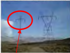
Figure 1-8. Left powerline: The Pacific Direct Current Intertie (PDCE), near Bishop, CA. HVDC, 3,000 MW, +/- 500 kv bipole, 844 miles from Cabo, at The Dalles Dam, OR to Yubaar (NW Los Angeles, CA). Commissioned in 1979 as 1,500 MW line. The right powerline is conventional high voltage AC.
