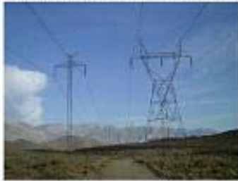
Figure 1-8. Left powerline: The Pacific Direct Current Inter tie (PDCI), near Blythe, CA. HVDC, 3,000 MW, +/- 500 kV bipole, 546 miles from Collins, at The Dalles Dam, OR to Sylmar (NW Los Angeles, CA). Commissioned in 1970 as 1,500 MW line. The right powerline is conventional high voltage AC.
