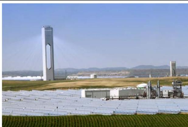
**Figure 4: Concentrated solar systems: trough collectors in front line, tower behind** (Source: Abengoa)
