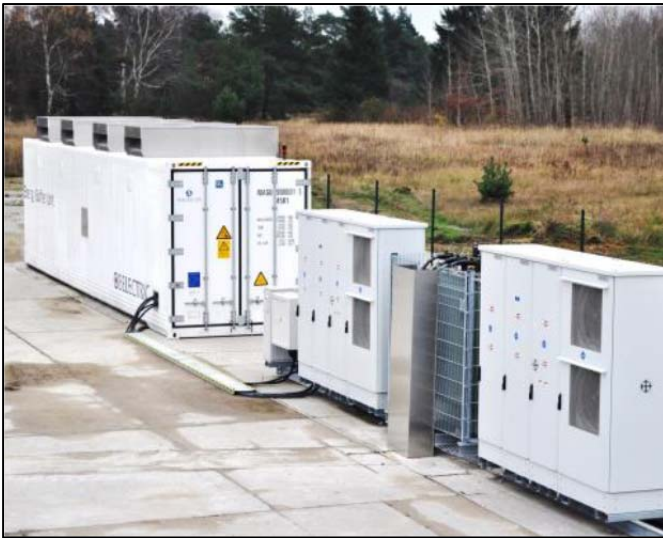
Figure 27 Belectric 948 kWh storage facility at solar power plant Alt Daber, Germany
